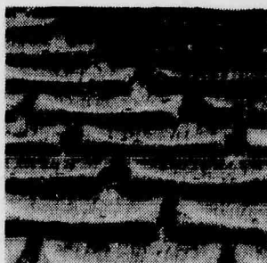
Problem: Damaged shingles.
